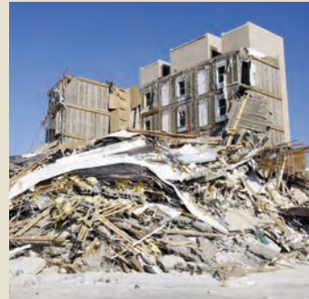
AFTER IVAN A hurricane-damaged condo in Alabama
